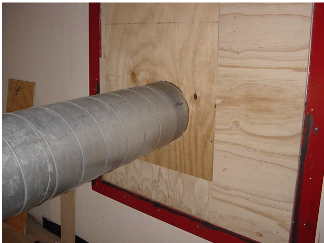
Photo B2: Rigid Duct Fitted to Transition / Spigot which Penetrates in to the Reverberation Test Chamber
